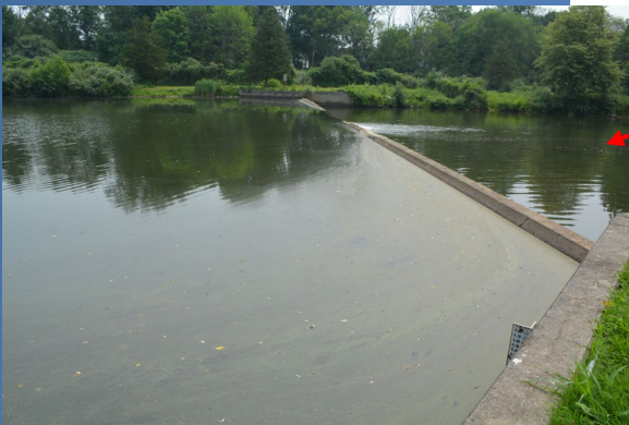
Spruce Run Outlet, July 20, 2021 Source: NJWSA
