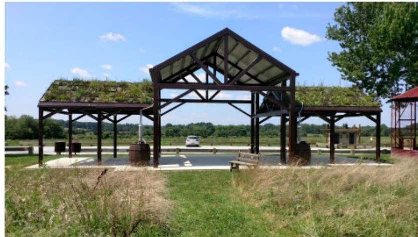
Rain Barrel Irrigation at Mercer Meadows
